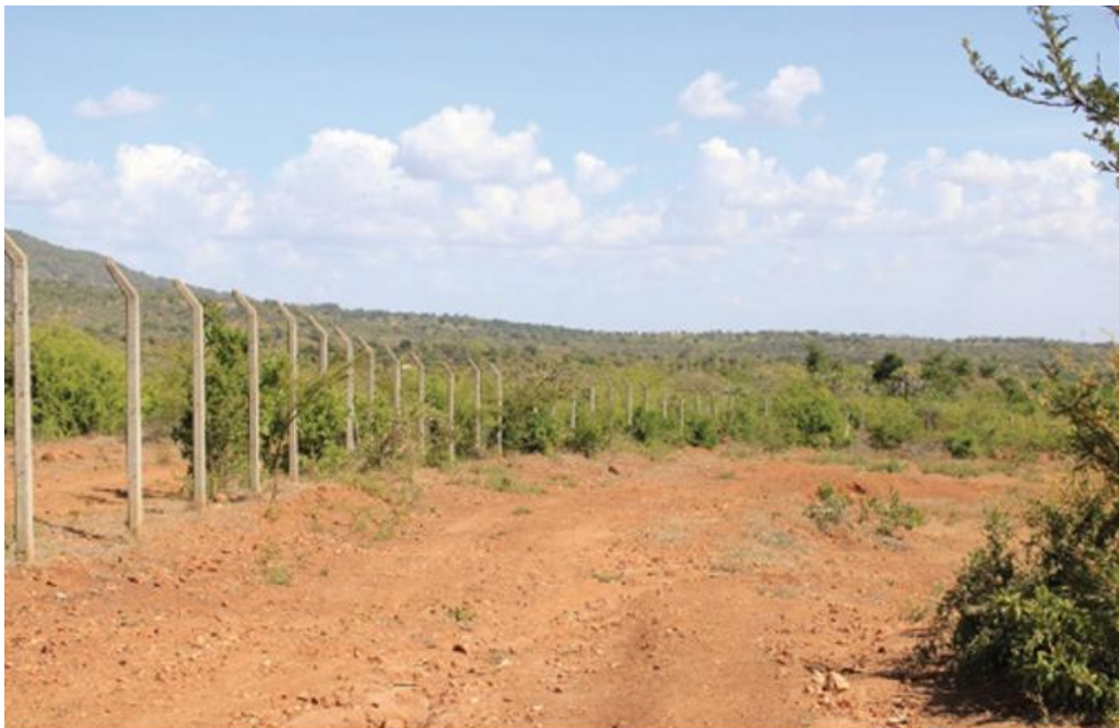
Figure 2-13: Kamwimbi Landfill Perimeter Wall
