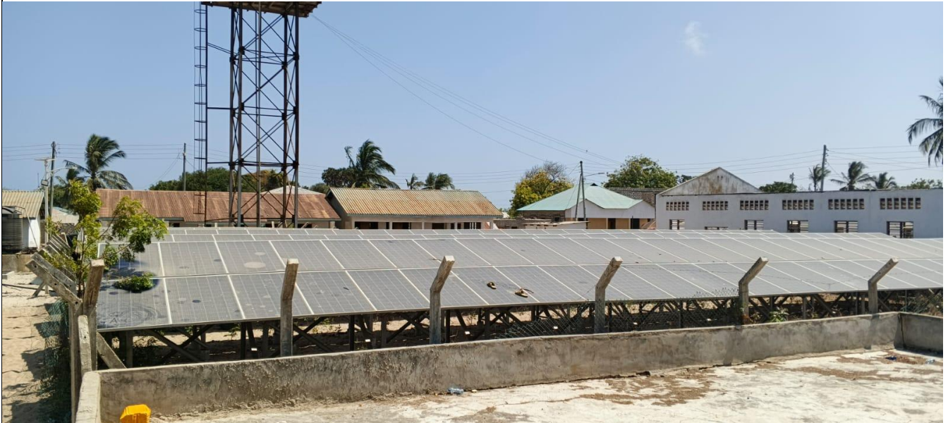
Figure 1 The Kiunga Solar Desalination and Community Water Governance Initiative in Lamu County, featuring the solar panels that power the water supply system.
