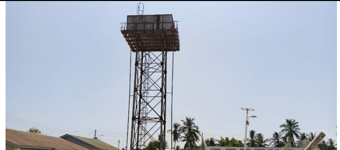
Figure 12 One of the tanks used for water storage
