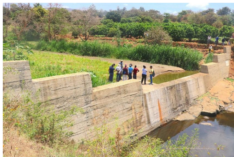
Figure 3 One of three sand dams constructed to provide reliable water sources for over 500 farms and households
