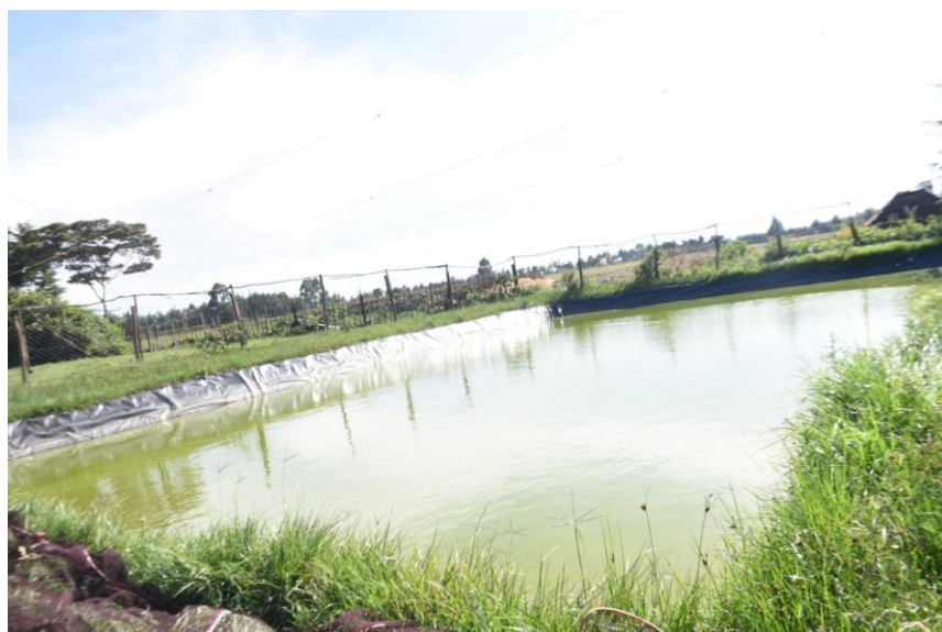
Figure 2: A lined earthen pond at Sila Bore's farm in Sergoit Ward, Moiben Sub-County, designed to retain water and enhance fish production in drought-prone areas.
