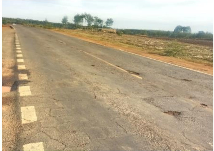
Plate 84: Kitale-Eldoret Road with potholes (Source: Simuplan fieldwork 2019)
