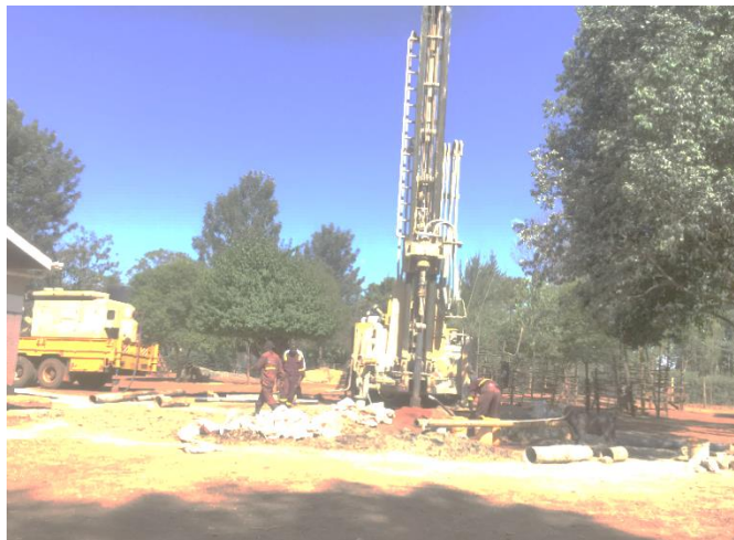
Plate 118: Borehole drilling (Source: Simuplan, 2020)
