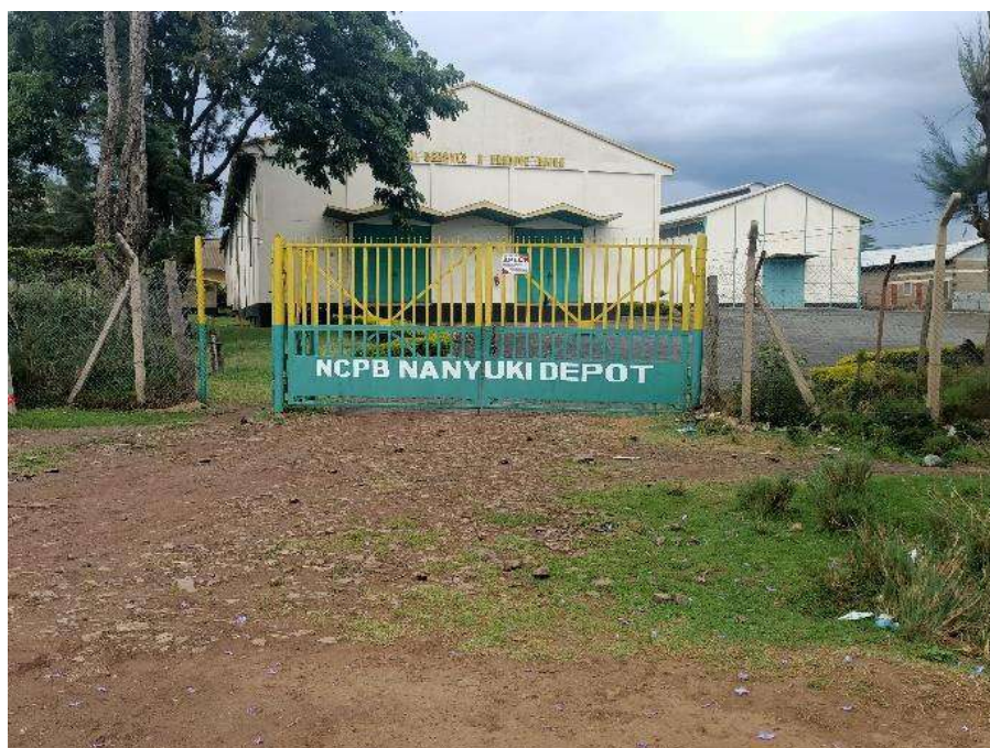
Plate 8-2: Grain Warehouses at Nanyuki and Ol Moran
