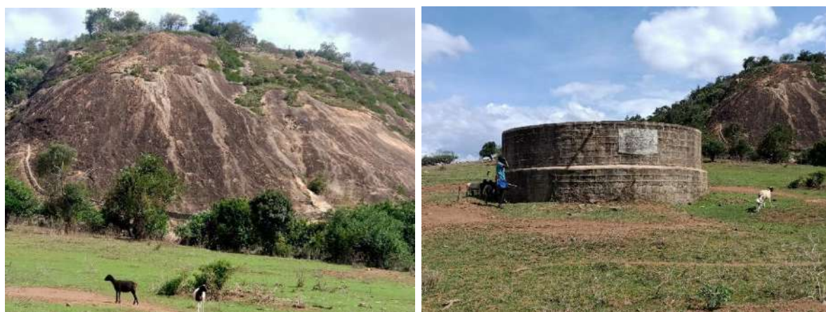
Plate 9-8: A Rock Catchment and Community Storage Tank
