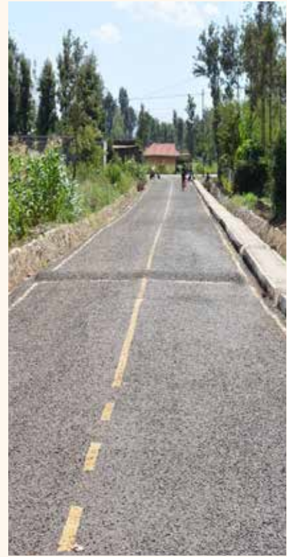
Completed Kabati Road with Markings, Side walk and drainage
