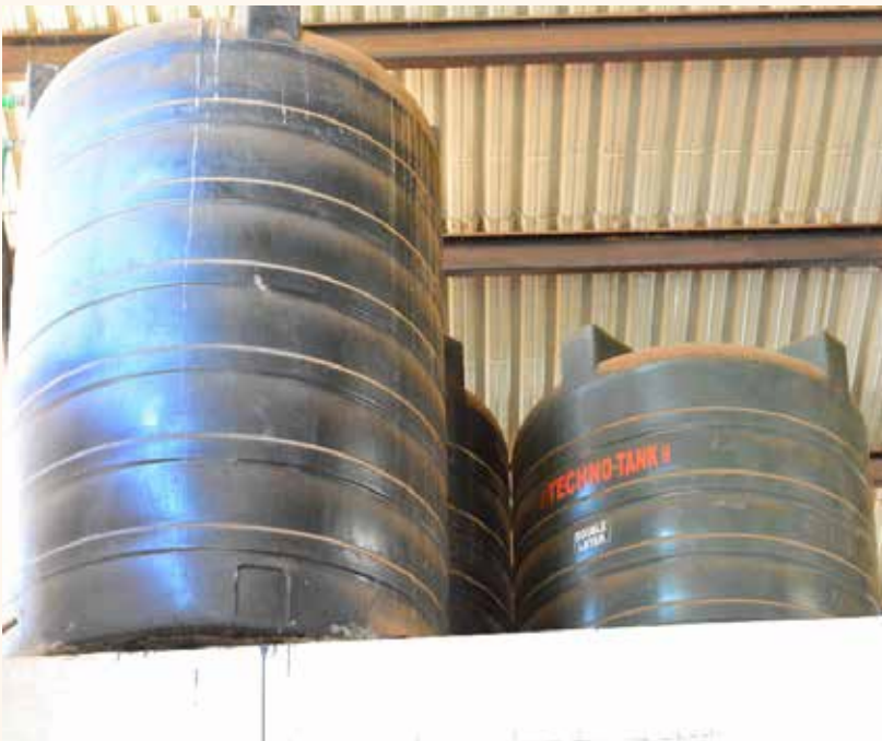
Water tanks for water provision and storage used for cleaning of the market as well as the toilets
