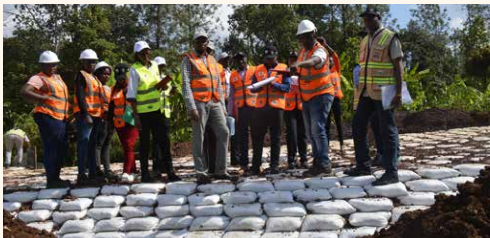
A photo of 'Do-nou' arranged in grid patterns awaiting topping with appropriate surfacing material
