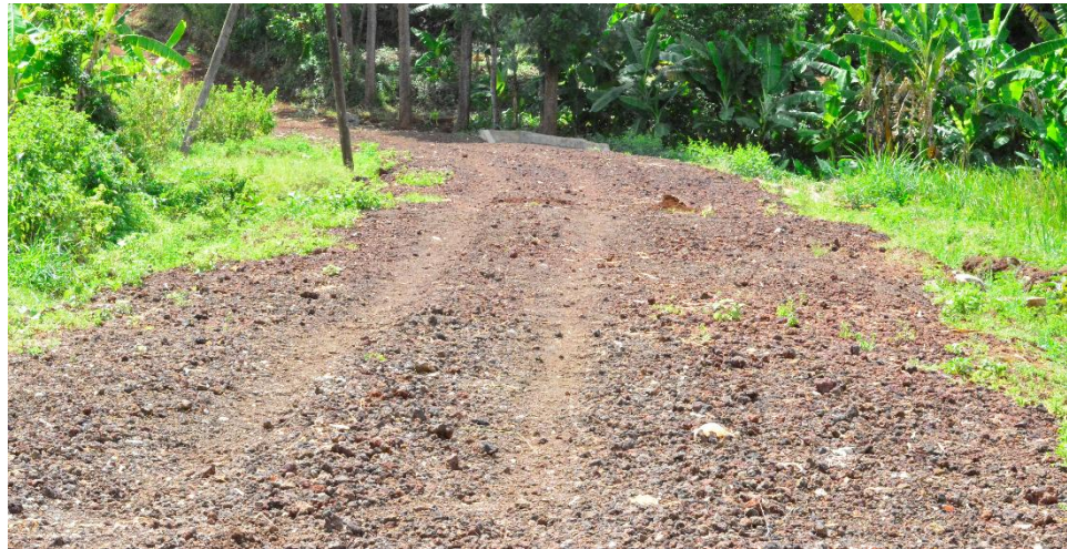
A completed road section maintained using "Do-nou" technology
