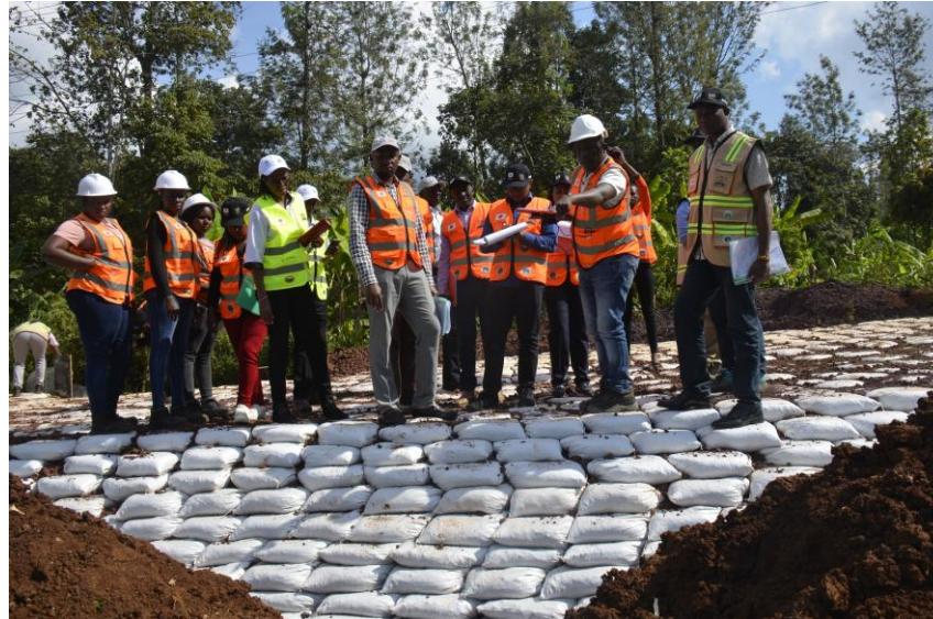
A photo of 'Do-nou' arranged in grid patterns awaiting topping with appropriate surfacing material
