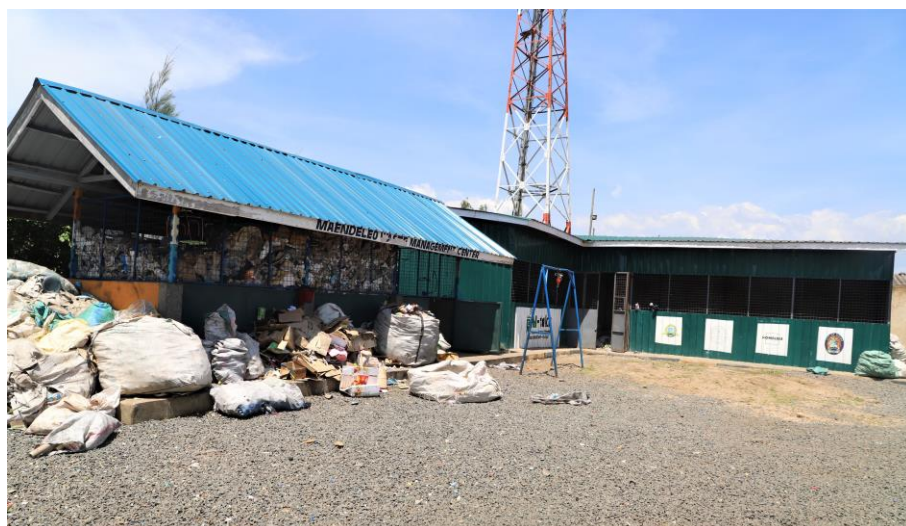
A photo of the Maendeleo Waste Recovery Center
