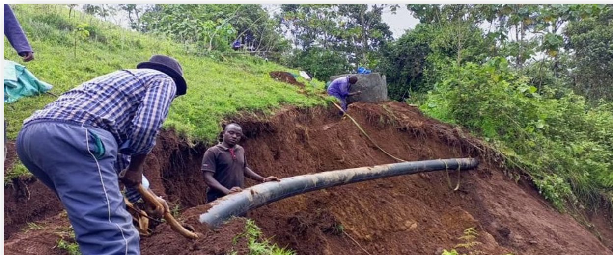
Figure 12: Community Members Anchoring a pipeline exposed by a landslide
