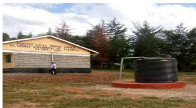
Two ECDE classrooms, two stores and an Office done by World Vision
