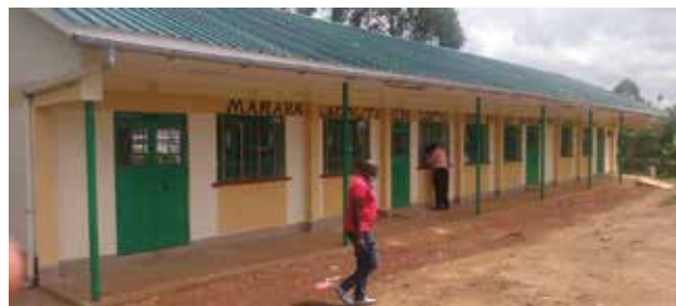
Three ECDE classrooms, two stores and an office at Maraba ECDE Centre, Lurambi Sub-county, Kakamega County
