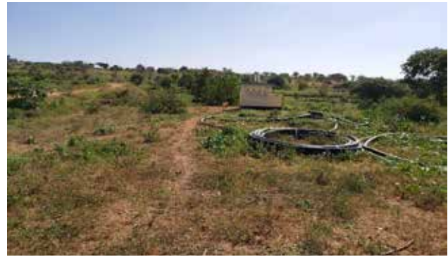
Leftover piping material at the Kwa Mbila Dam & the toilet in the background with project information
