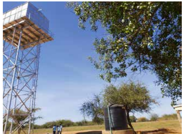
An elevated water tank, a ground tank and a water kiosk partly hidden
