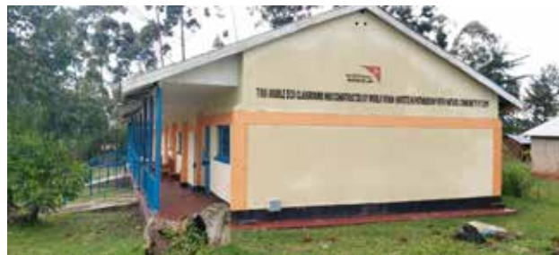
Two ECDE classrooms, two stores and an Office done by World Vision
